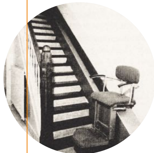
Our first seated stairlift is installed
