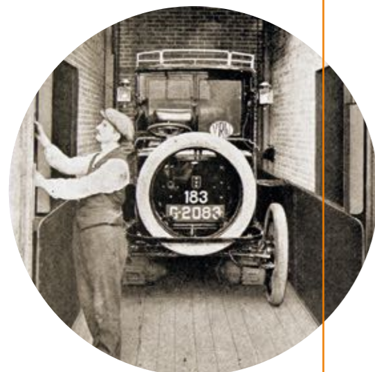
In just 4 years, we installed over 600 lifts
